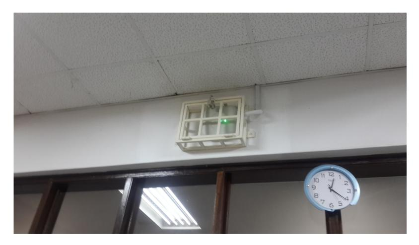
In this case, physical security interferes with the correct operation of the wireless AP.
